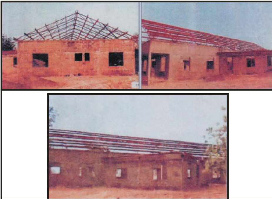
Church building at Rafter Level.
